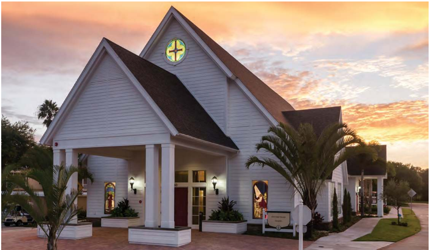
The Chapel at Sunnyside Village.
