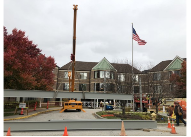
First steel columns being placed for porte-cochere
