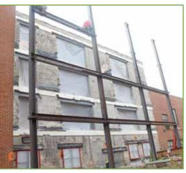
New exterior foundation installed for new wall structure.
