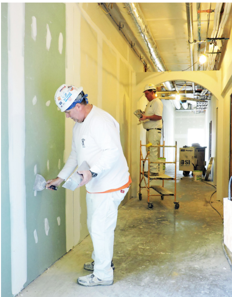
Tradesmen mud drywall and install doors and trim in the new Village II building.
