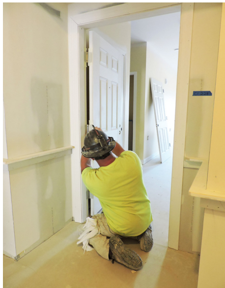
Tradesmen mud drywall and install doors and trim in the new Village II building.
